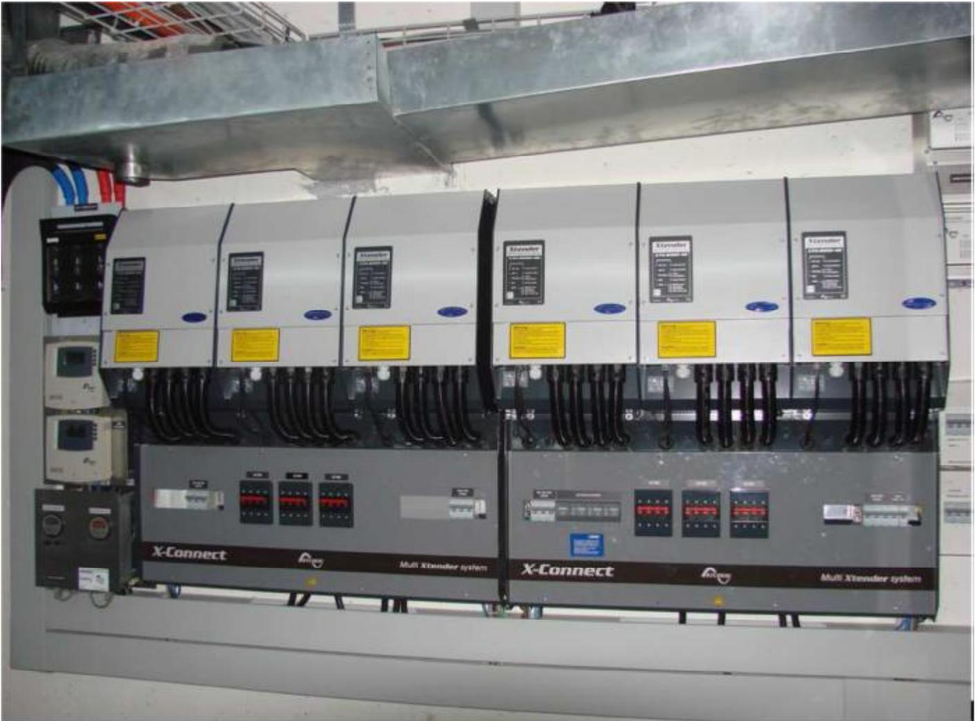
Each inverter has a nominal power of 7kW and can also emit 8kW for 30mins. But an emission of peak current of 21kW for 5 sec. is possible, too. This involves that 6 inverters together give off a continuous output of 42kW and for the short time the car elevators start releases up to 126kW safely.
