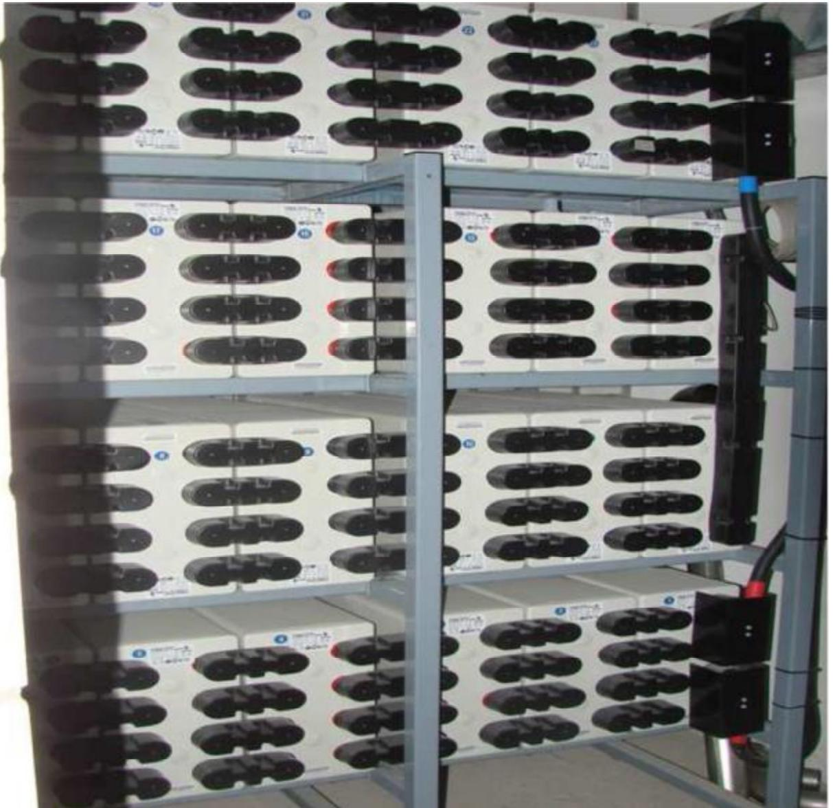
This battery of the type 2 CP 3'000 has a nominal tension of 2 Volt. With this system 24 pieces in series are being switched on resulting a 48V-Battery with a capacity of 3'000 Ah.
