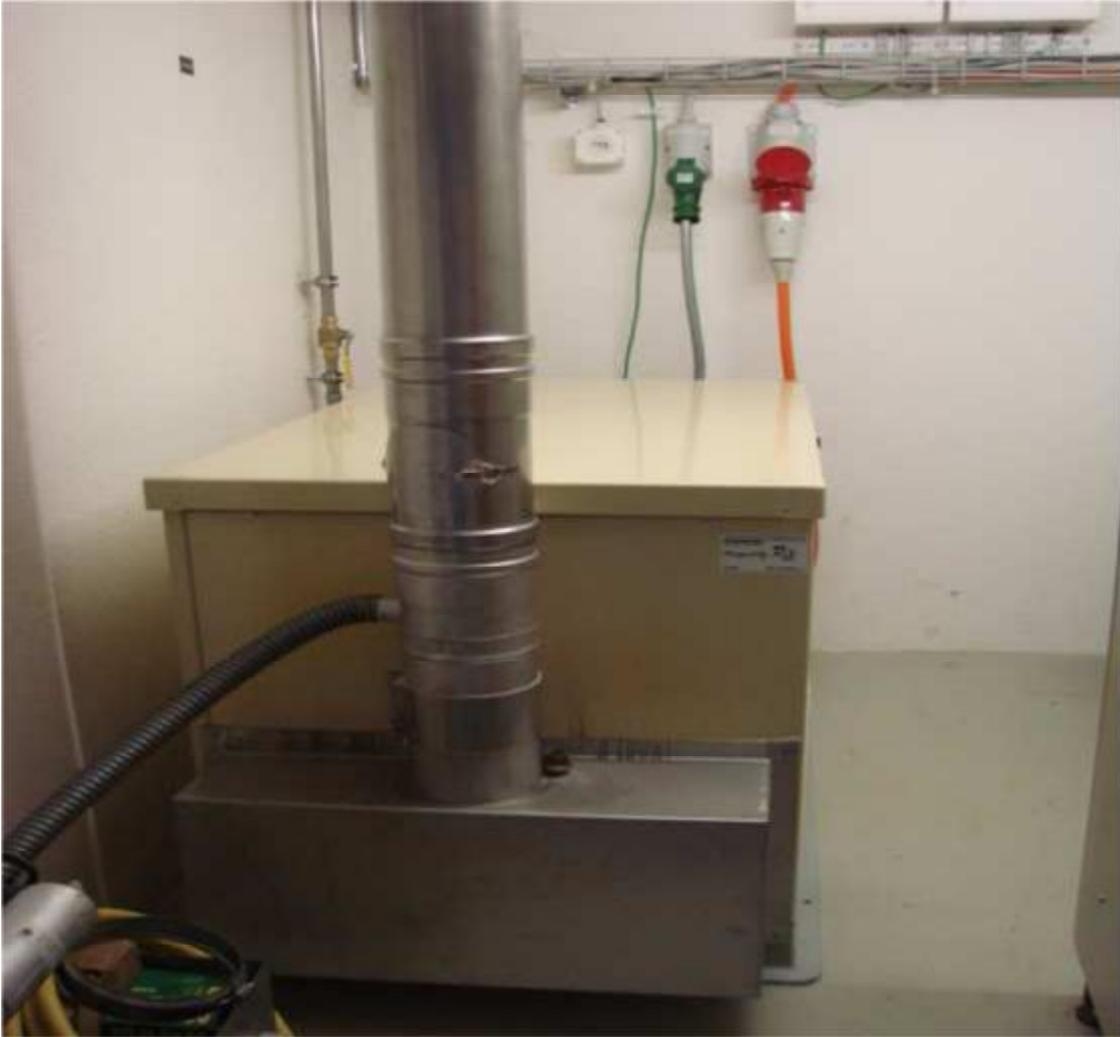
The emergency generator has a max. power of 9,3kW a gas consumption of ca. 3,6 kg/h and an overall efficiency of ca. 90%.
